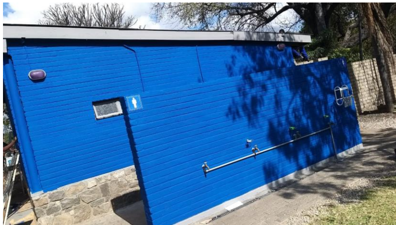
New-look change rooms by the swimming pool
